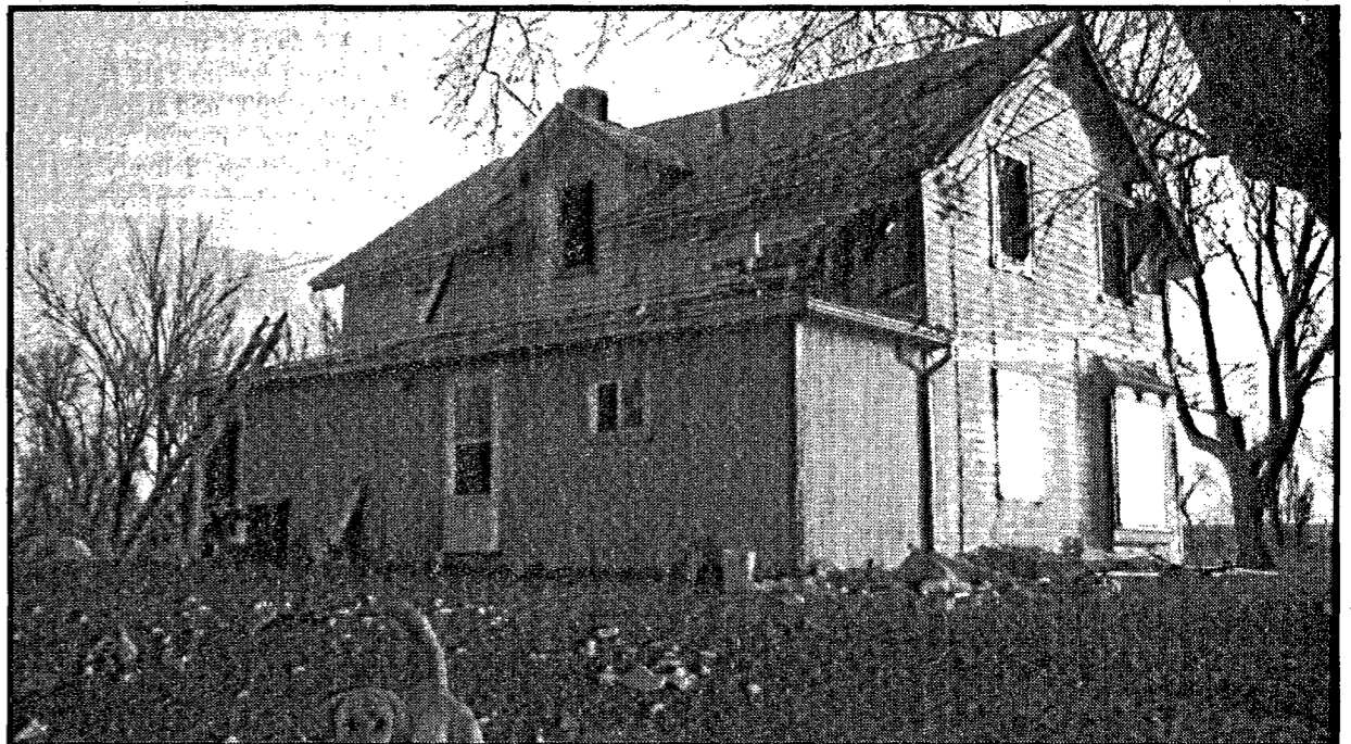
The home of Duane and Kim Nelson of rural Dixon was destroyed following a fire last week. No one was injured in the blaze.
